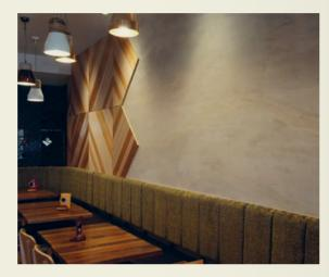
Natural renders are often thought of as a traditional building material, but Rockcote, a New Zealand-owned company that manufactures earthen renders from clay and lime, has rethought the application for contemporary use.
