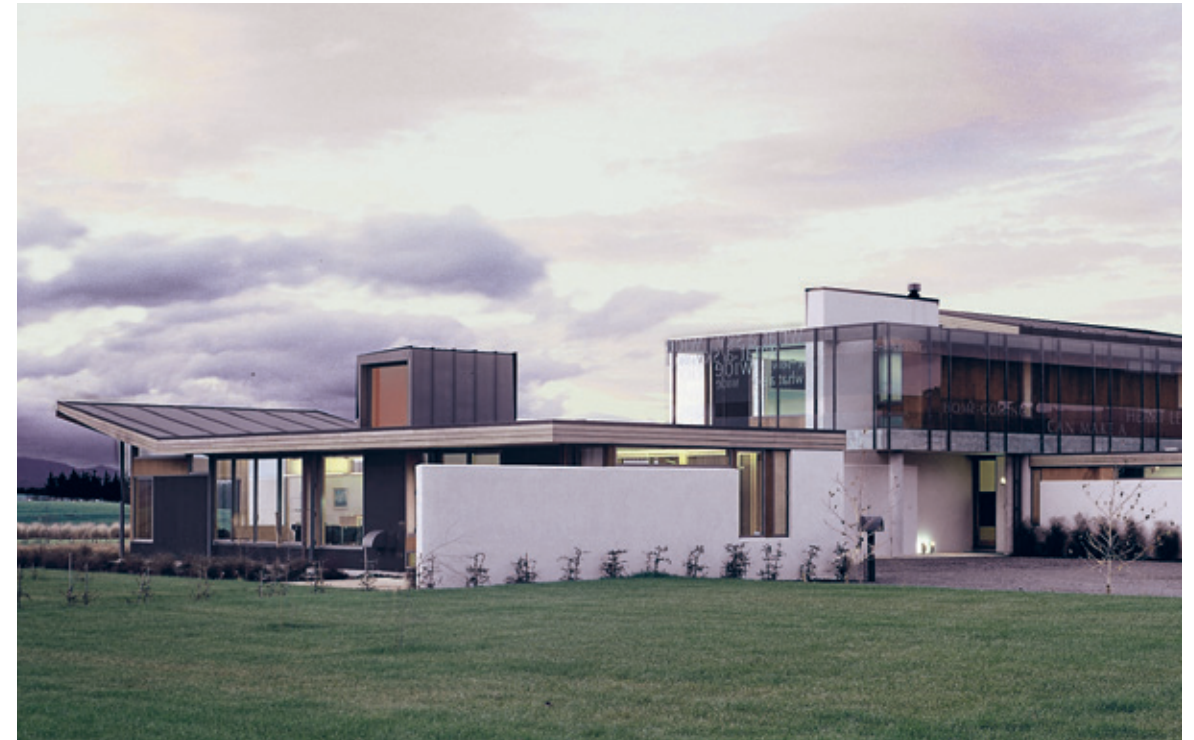
Below: Ponatahi House, view to north.
