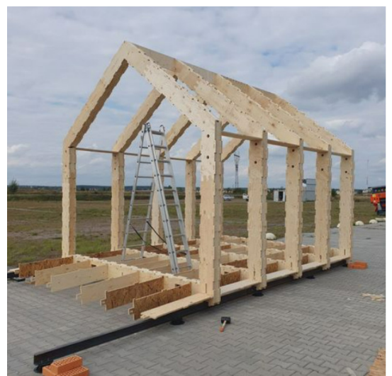
Fig.45. Structural components of a WikiHouse.
