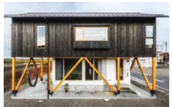
Fig.9. Ushijima Architect's small wood-clad house, raised on a concrete base to help mitigate the risk of flooding.
