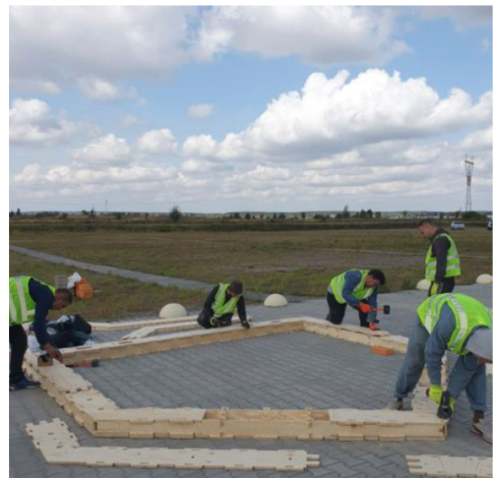
Fig.44. On-site assembly of a WikiHouse.
