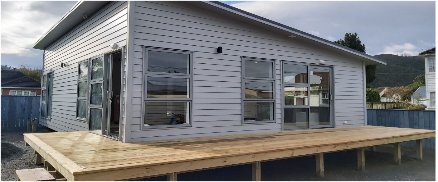
Fig.46. EasyBuild home built on elevated timber piles.
