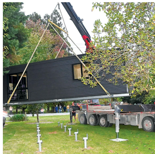
Fig.28. Relocatable housing pods being installed on site in Tairāwhiti.
