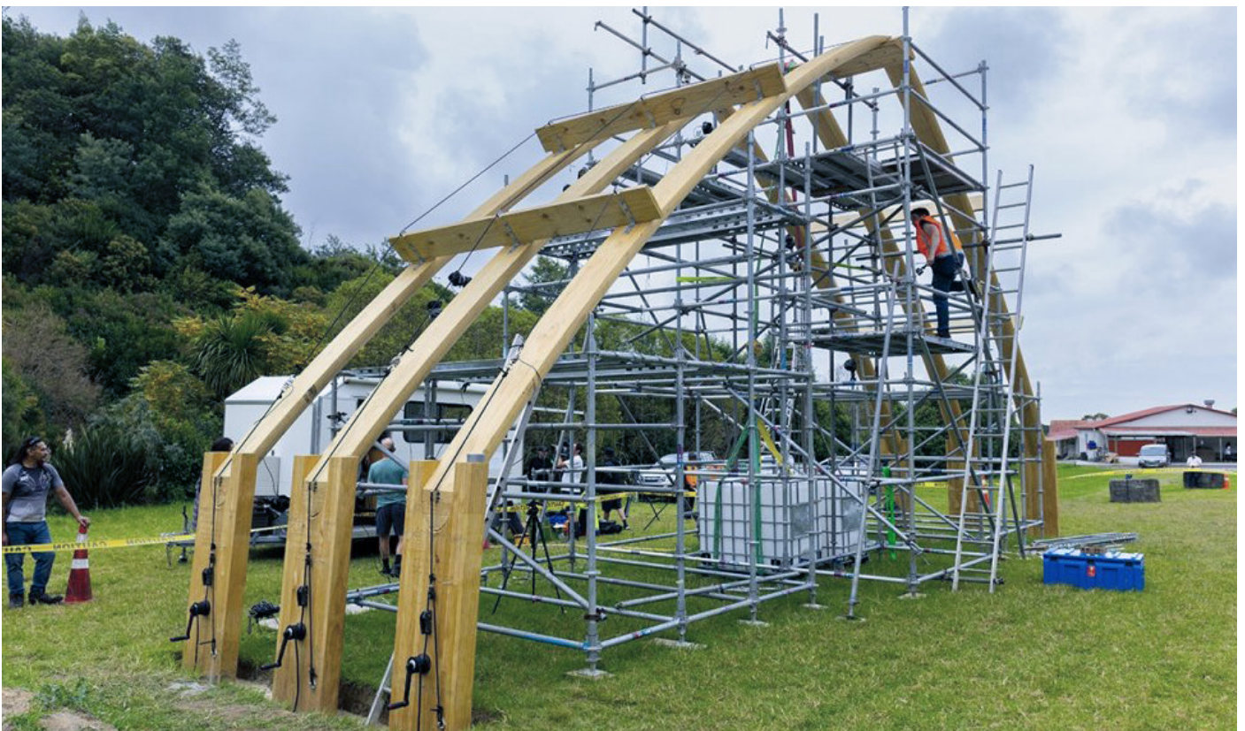
Fig.33. An endangered construction technique called 'mīmiro', where timber portals use interlocking compression joints, instead of bolting parts together. EQC. (n.d.).
