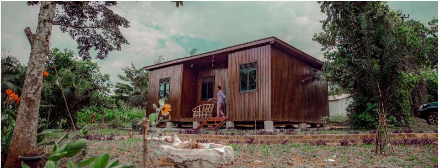
Fig.37. First Easy Housing three bedroom 50 sqm home on concrete piles.
