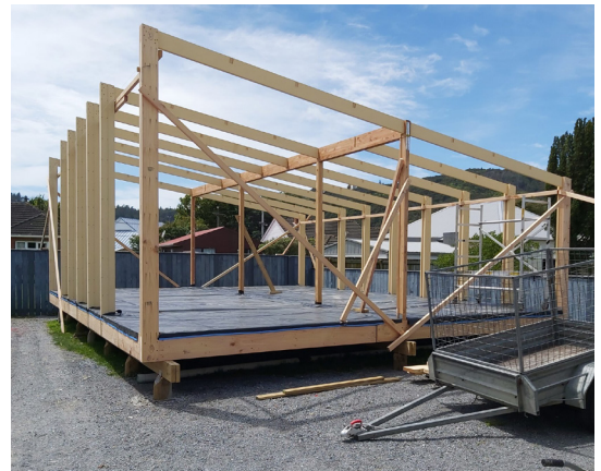
Fig.47. Construction of EasyBuild home using its modular framing system.
