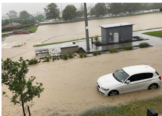
Fig.10. Greenslade Reserve in Northcote Development is a stormwater detention basin as well as a sports ground and park. It collects water and redirects it away from homes.
