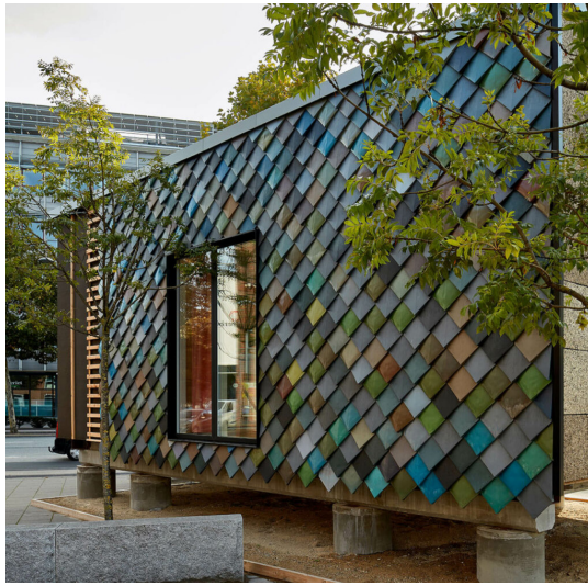
Fig.23. Circle House's recycled material facade.
